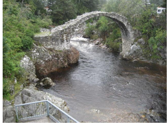
Ruined bridge at Carrbridge
